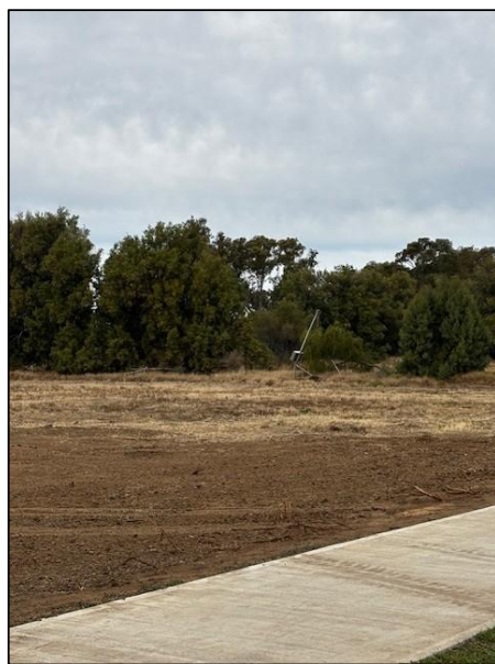
Figure 5: Cleared site with utility connection in background
