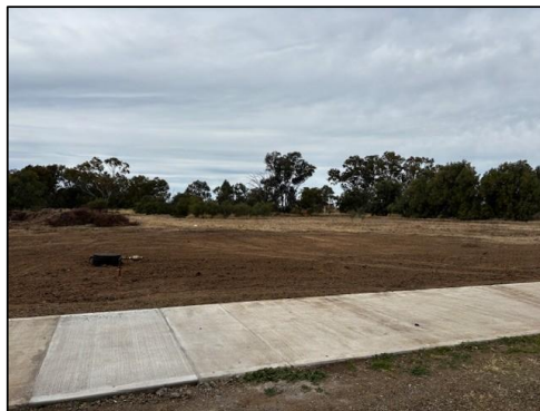
Figure 3: Site looking east from Calga St. New footpath in foreground
